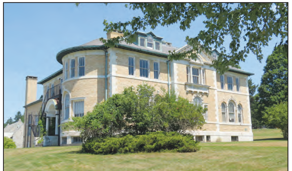
A new Planning Committee must solve the challenges of the deteriorating Thorne Memorial Building in Millbrook. Photo by Curtis Schmidt
